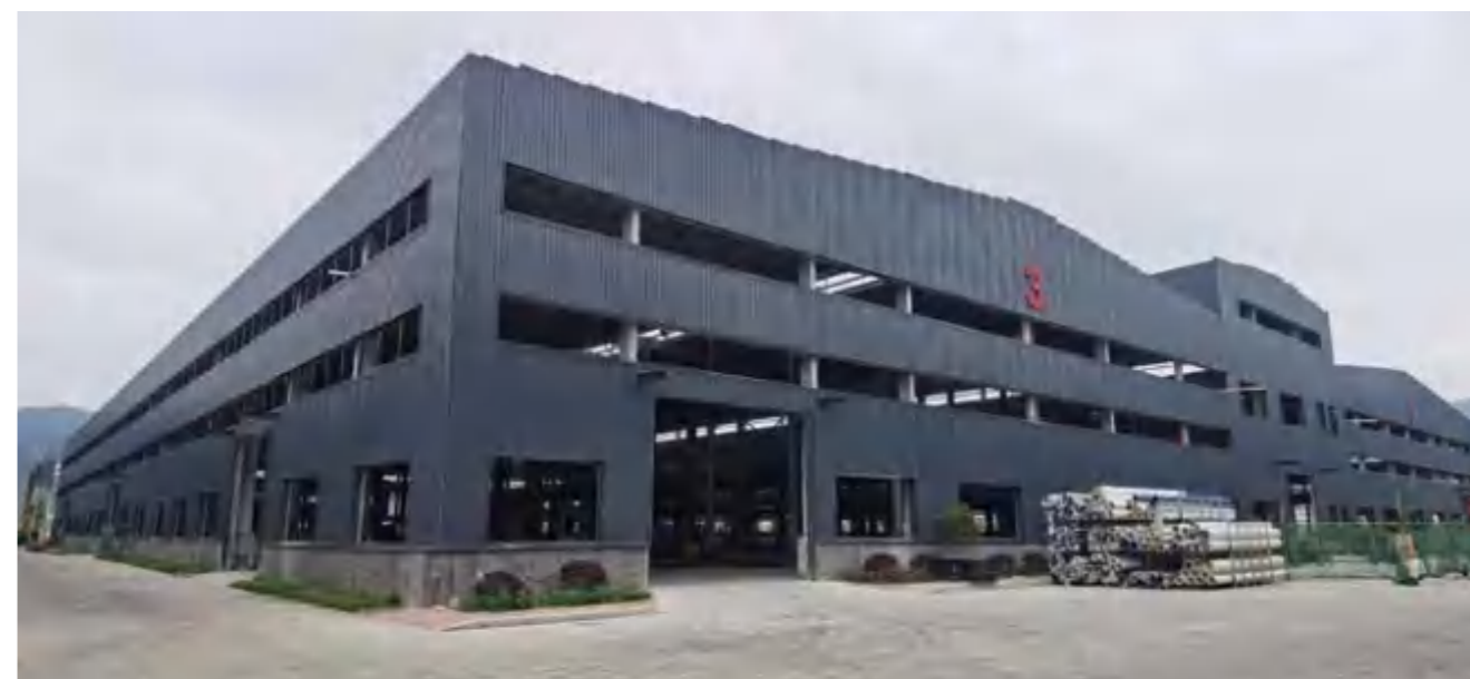
Fujian Lesso New Material Technology Co., Ltd. Phase I Plant Project
