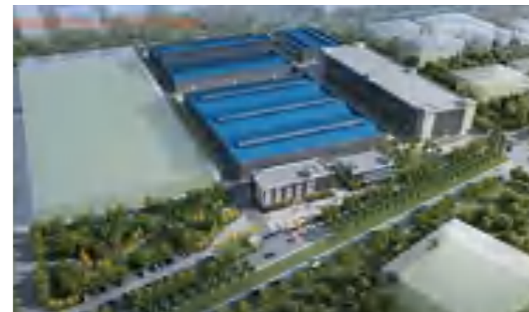
Project: Indonesia Lesso Factory Work Scope: 3 Factories Site area: 37,230 m 2 Lead time: Feb, 2021
