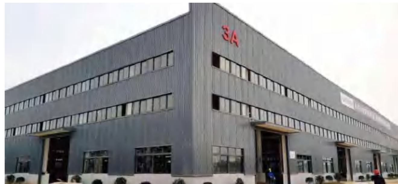
Jiangxi Nanchang Lesso Technology Co., Ltd. project
