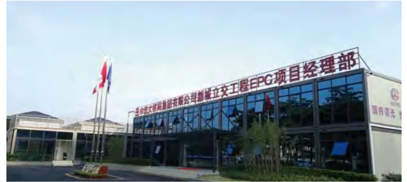
Manager Department, EPC Project of New City Interchange, by China Railway Bridge Bureau Group Sixth Engineering Co., Ltd.
